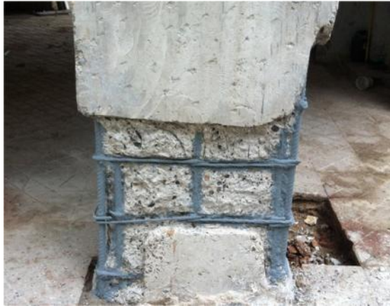
TYPICAL IMAGE OF SURFACE PREPARED RCC MEMBER
